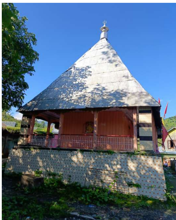
Renovated temple at Panyalag.
